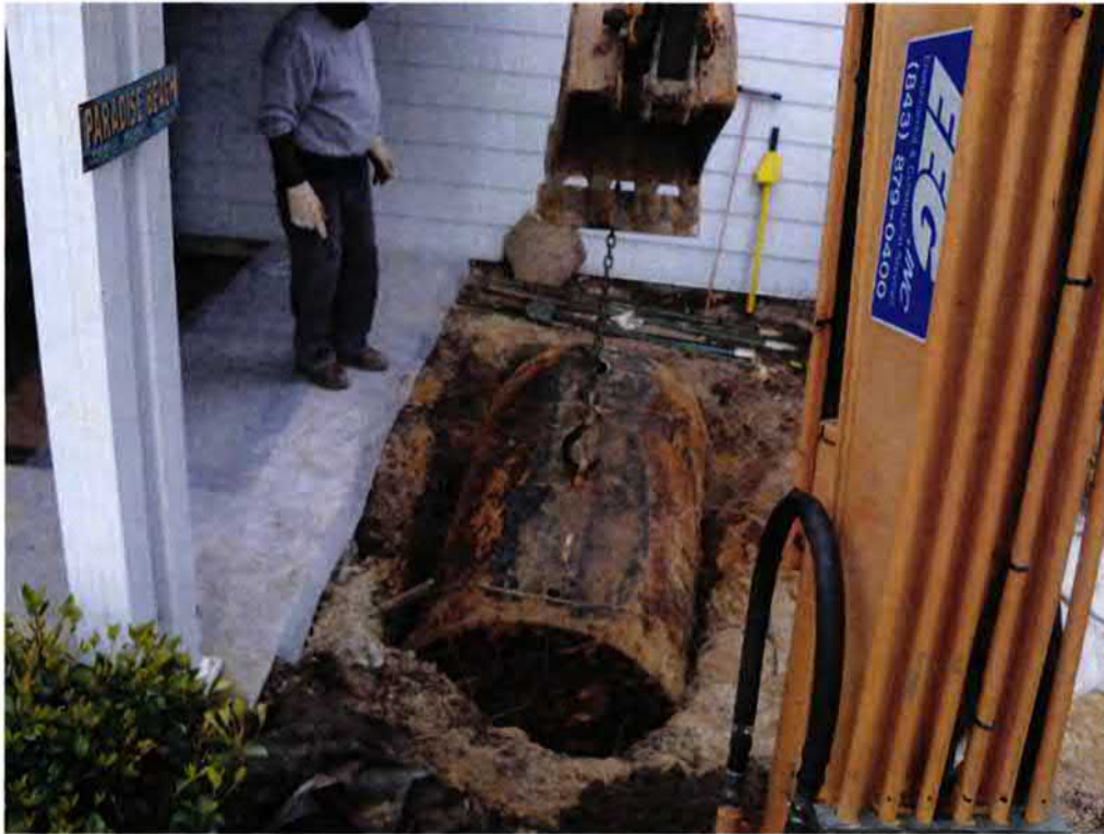
Picture 3: UST 372Aspen-2 being removed.
